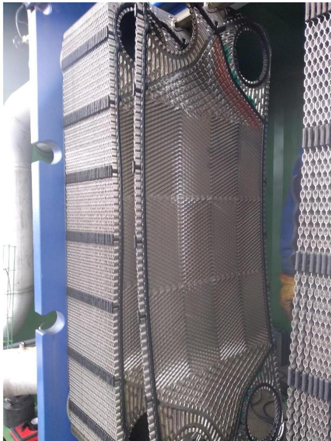
Figure 6: A laser welded module "sandwich" heat exchanger plate within a semi-welded heat exchanger being disassembled.
