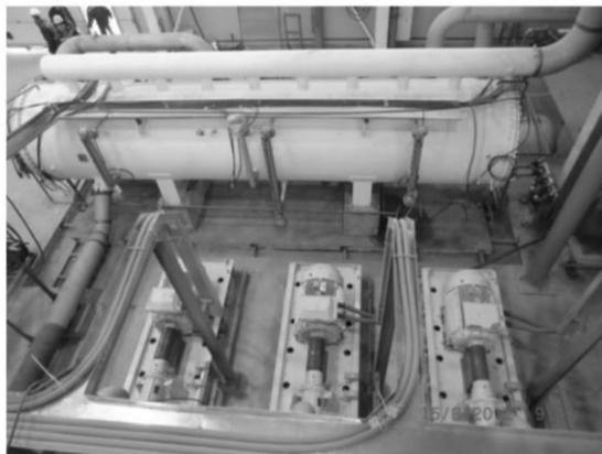
**Figure 22:** Evaporator type vapor superheater used in the Pauzhet GeoPS binary power unit with a cluster of feed pumps.
