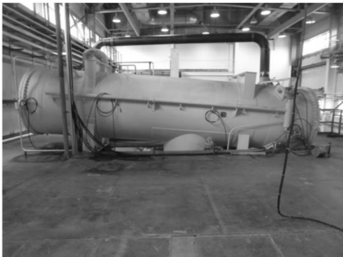
Figure 25: Condenser of the binary turbine unit at the Pauzhet GeoPS.
