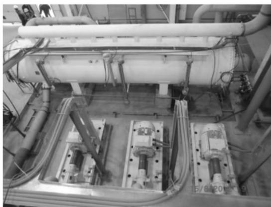
**Figure 22:** Evaporator type vapor superheater used in the Pauzhet GeoPS binary power unit with a cluster of feed pumps.
